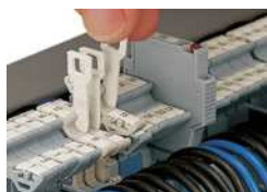
Pulling a disconnect tab.
